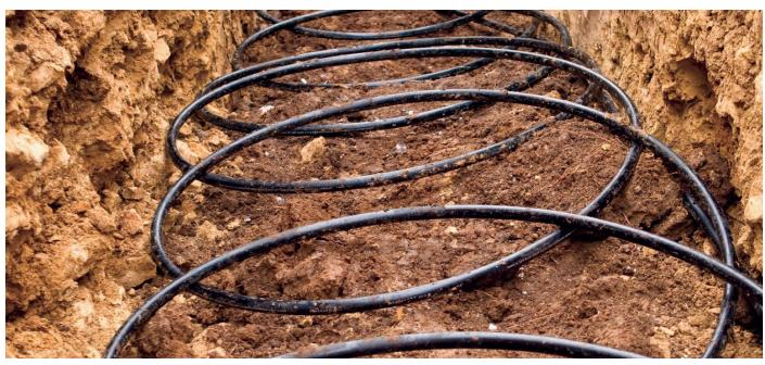
**Geothermal coils:** Approximately two and a half metres underground, this coil serves as part of a geothermal system enabled by Dow technology to heat and cool homes, schools and businesses.
