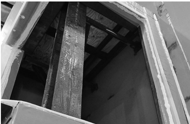
Figure 7: DOWSIL™ Silicone Transition system-wrapped opening
