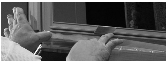
Figure 13: Folding strip onto mullion and attaching with sealant
