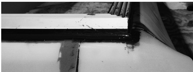
Figure 2: Corner and strip pieces installed in-shop
