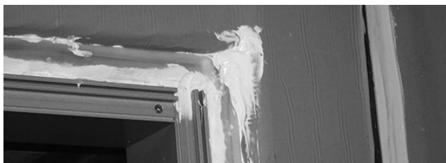
Figure 12: Folded and sealed corner
