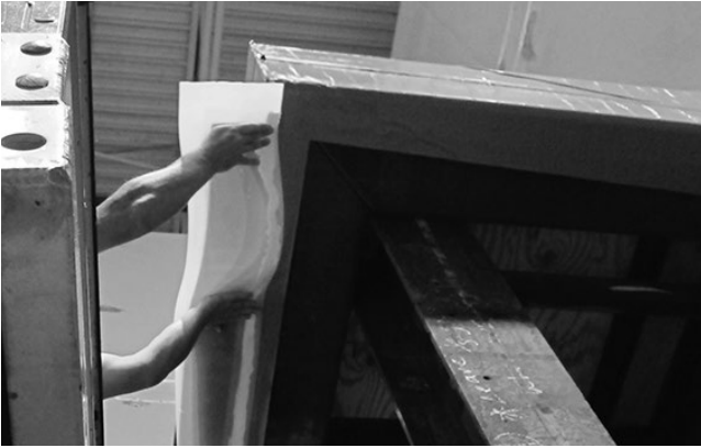
Figure 9: Installing strip at head of fenestration unit using sealant
