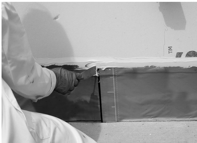
Example of bridging from below grade water proofing to Air Barrier using DOWSIL™ 758 Silicone Weather Barrier Sealant
