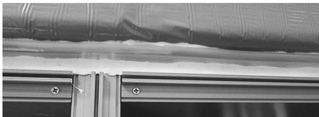
Figure 14: Finished strip installation
