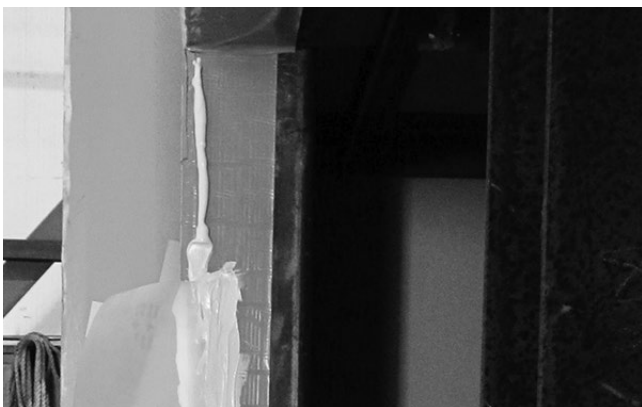
Figure 8: Keep splices a minimum of at least 12 inches (300 mm) from corner
