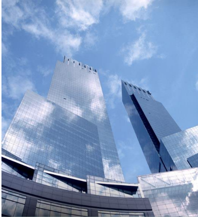
4-sided silicone structural glazing
