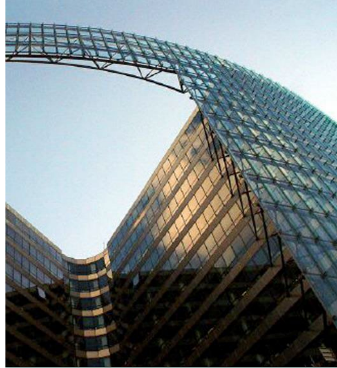
2-sided silicone structural glazing
