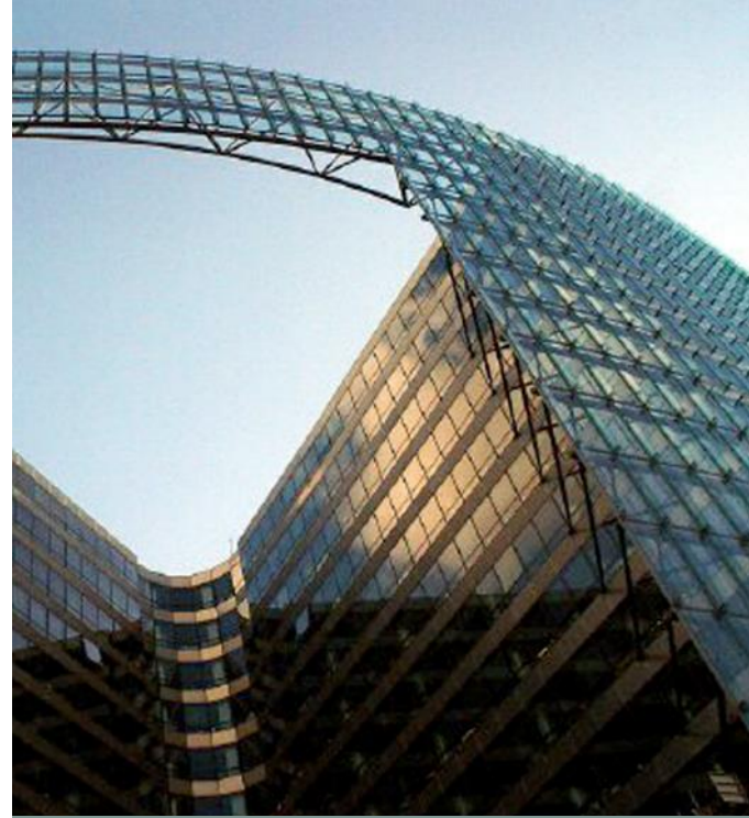
2-sided silicone structural glazing
