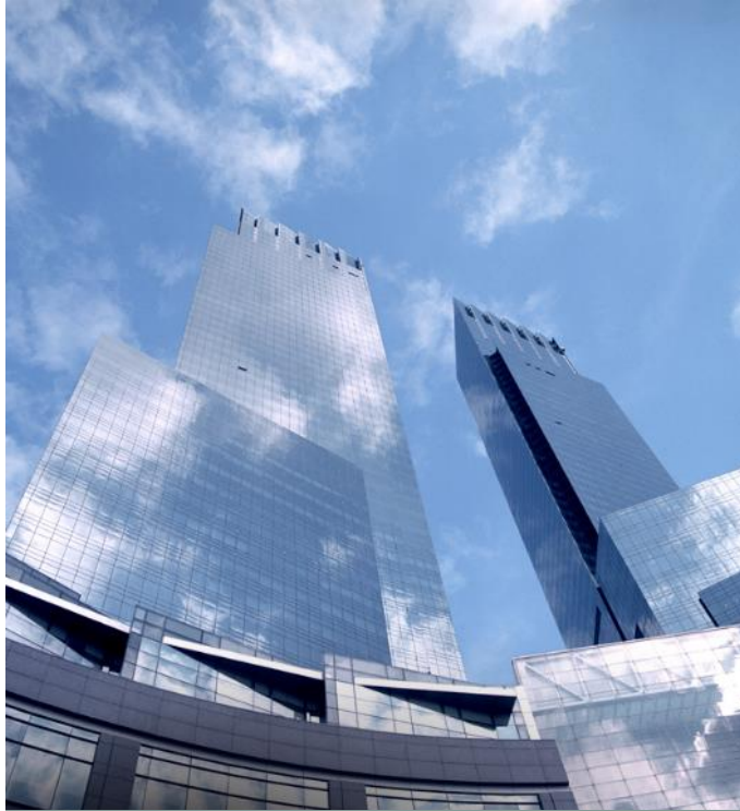
4-sided silicone structural glazing
