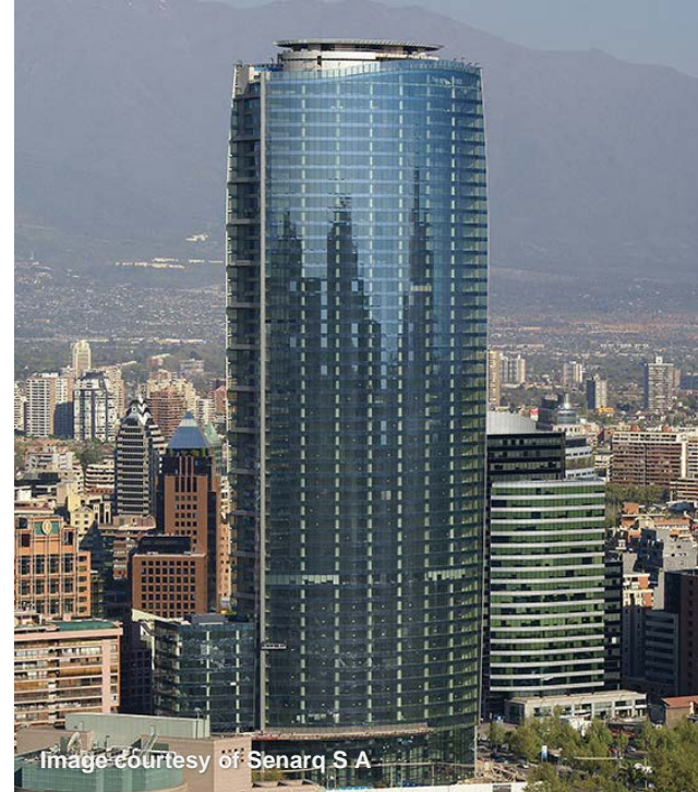
Torre Titanium La Portada in Santiago, Chile, survived an 8.8 earthquake without damage
