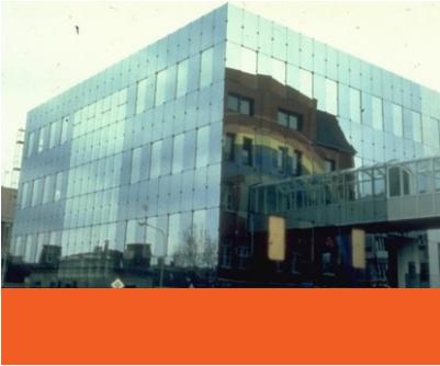
1987: Selb, Germany 4-sided SSG with safety devices
