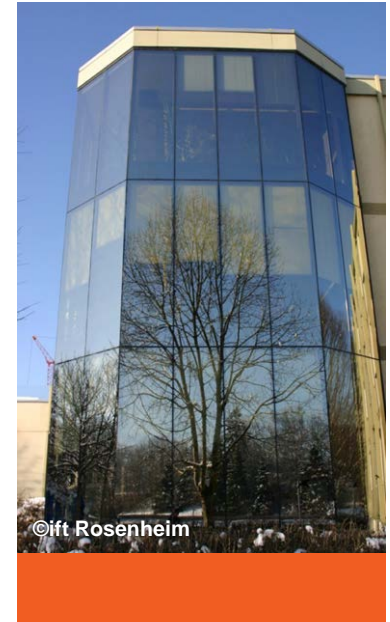
1985: Rosenheim, Germany ift Rosenheim; 4-sided insulating glass toggle system; no safety devices
